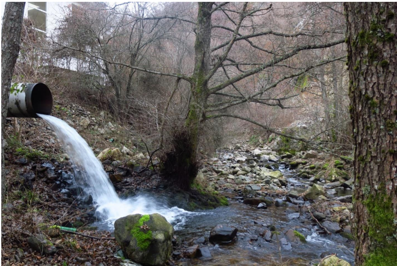
Discharge of water below Blagoevgradska Bistritsa-8 HPP not described in the EIA/AA screening decision, 21 December 2020
