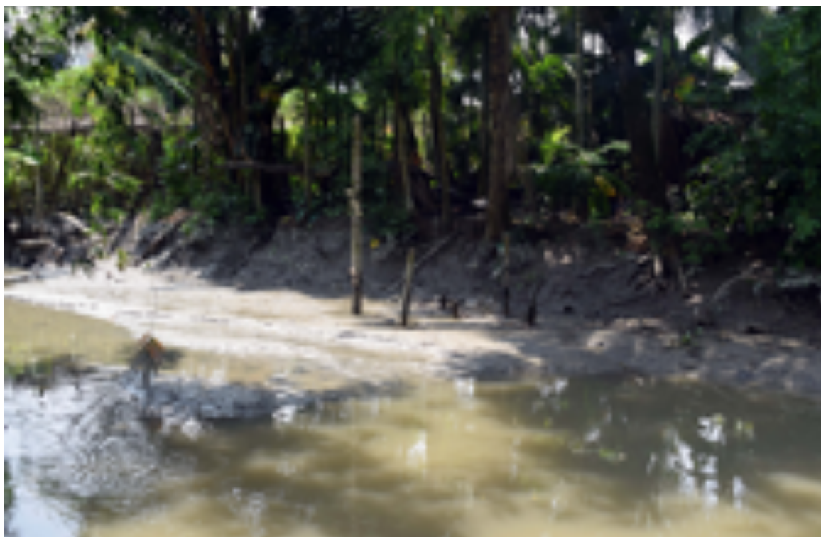
Figure 5. The NBBL embanked its northern part with sand sacks and has taken over half of the canal. The sand from the sacks has spilled out into the canal-bed causing siltation and the canal to gradually dry up.
