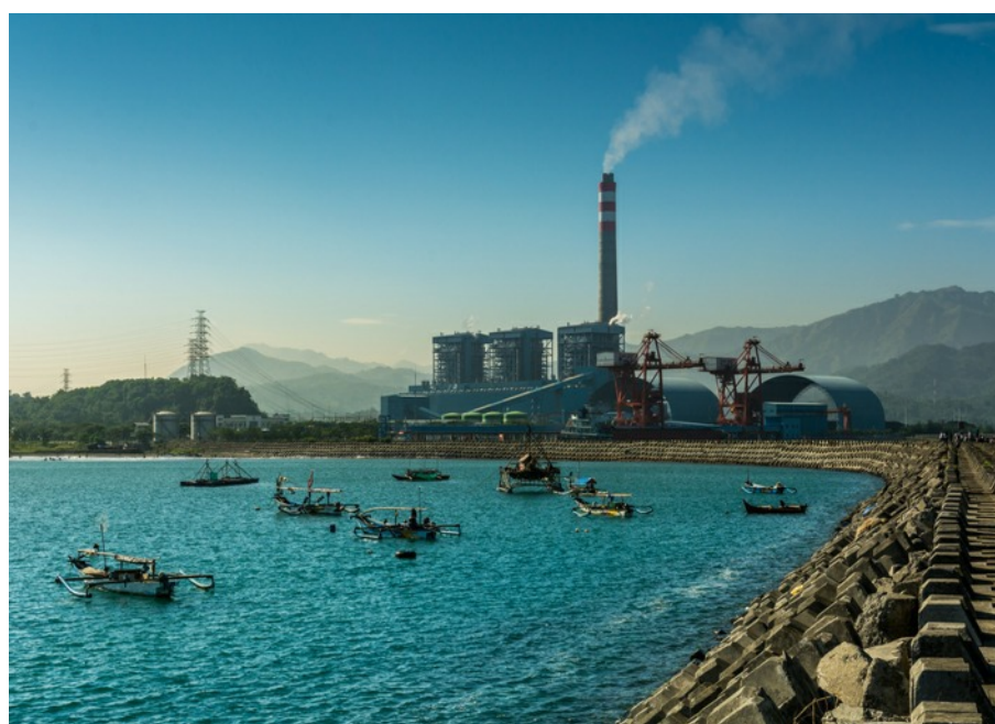
Photo: Coal Power Plant PT. Indonesia. Credit: Ares Jonekson/Shutterstock
