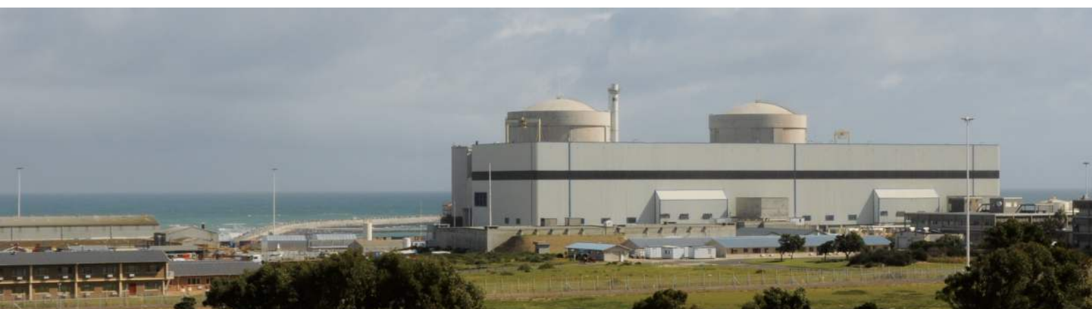
Koeberg nuclear power plant, Cape Town, South Africa. Photo by Paul Scott. CC BY-SA 2.0
