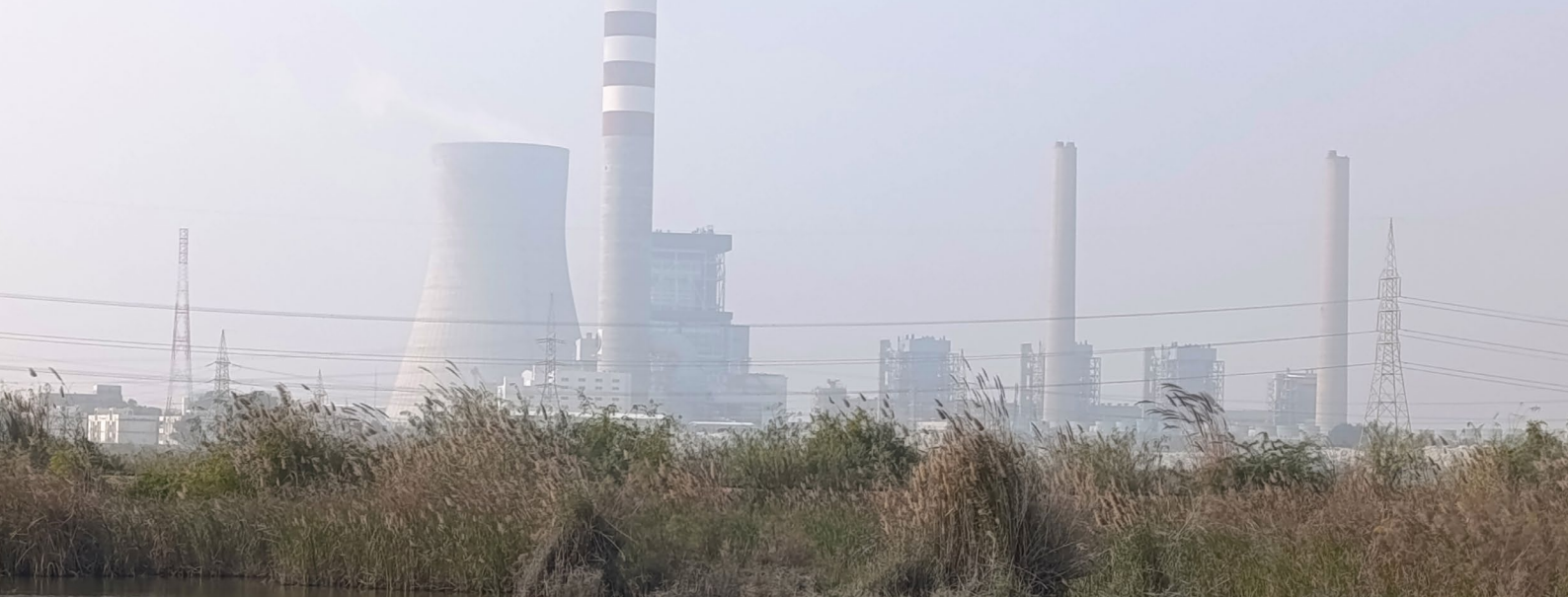
Jamshoro coal power plant. Photo by Alternative Law Collective.
